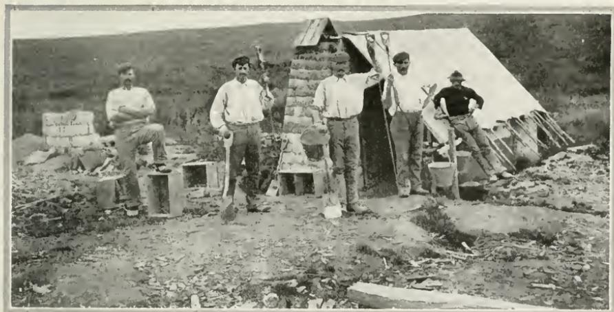
The best kauri gum is found ten or twelve feet below the surface of the ground, where ancient kauri forests are buried. The presence of the hidden treasure is determined by "spearing the ground." Long spearlike iron rods, such as are shown in the hands of the men in the photograph, are used to probe thru the soil and pipestone clay. Having located the gum in this manner, the diggers resort to pick and shovel. The picture shows a typical kauri gum diggers' camp.
