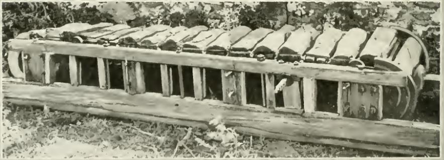
This treadmill, in the days when Tasmania was a penal colony, was used to turn a gristmill. It was operated by convicts and the heavy cleats are deeply grooved, having been worn down by the feet of the men who walked many weary miles on the machine without advancing.
