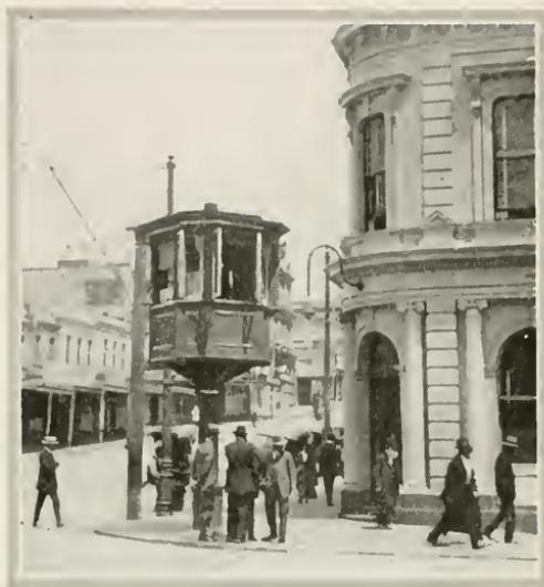
From this tower in the business section Auckland's street car traffic is controlled. All cars pass this tower, where a record of schedules is kept. Fares are charged according to distance traveled, lines being divided into sections over which passengers may ride for two cents a section. The longest ride in one direction is eight miles for twelve cents.
