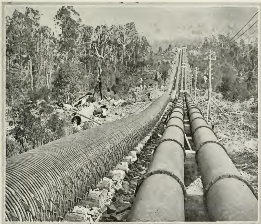
The pipes which carry the water from the Great Lake of Tasmania to the power house of the island's greatest hydro-electric development. The pipe on the left is of wood and was built during the war when steel could not be obtained. It is two miles long and forty-nine inches in diameter and is said to be the largest wooden pipe carrying water to a 400-foot head in the world. It is made of eucalyptus staves, held together by wire.
