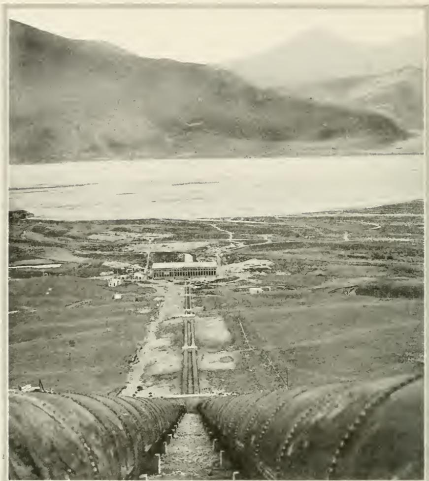
New Zealand is very rich in potential water power. In time her hydro-electric developments will make her independent of fuel. The picture shows the power house of the Lake Coleridge hydro-electric plant and the great pipes which carry the waters down the mountain from Lake Coleridge.
