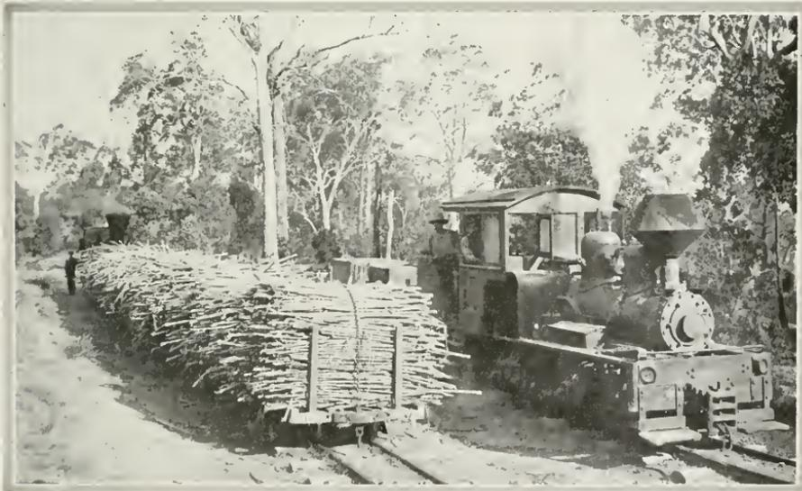
The State Railways' report asserts that Queensland owns thirty miles of "narrow gauge" railway. Elsewhere in the world a railroad three feet six inches in gauge is standard narrow gauge. That is the widest gauge in Queensland and the narrow gauge lines are two feet wide. For the most part, they operate in the sugar cane districts, where diminutive engines pull low trucks loaded with cane from the fields to the mills.
