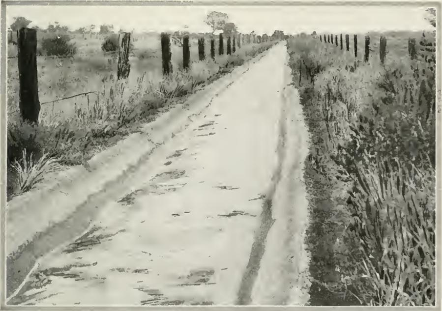
Hundreds of miles of these concrete-lined channels carry the waters of the Murray, longest river in Australia, into the arid lands which otherwise would not be productive because of the scant rainfall. This channel is part of the extensive irrigation system in the Berri district, noted for its splendid fruit. The state, which is back of all irrigation projects, builds dams and reservoirs and digs channels, and charges settlers for water equaling twenty-four inches of rain a year.
