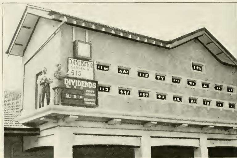
This is a photograph of the totalisator scoreboard. Under each slot is the number of the horse, and the figures in the windows indicate the amount "invested," or bet on the horse. The window at the top, near the roof, shows the total amount put up on the race, while at the left is a board showing the dividends which the winners pay. The "tote," as it is called, is the invention of a New Zealander.
