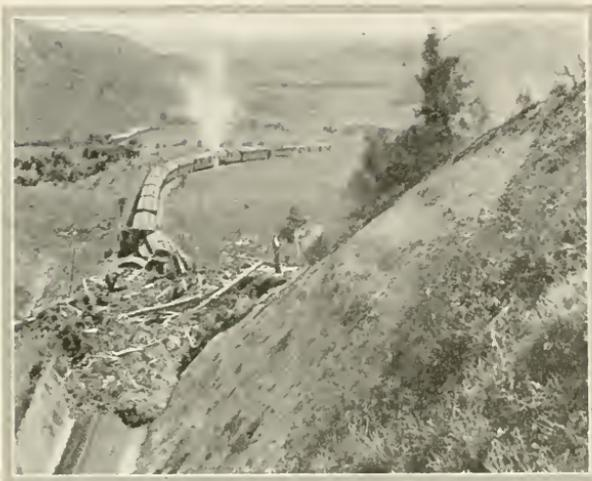
Accidents will happen on the best of railways. This is the most common kind of accident on New Zealand roads. In the hills and mountains earth and rock slides frequently block the rails. This passenger train came along just in time to be caught in a slide. The engine and two coaches were derailed, but there were no casualties.
